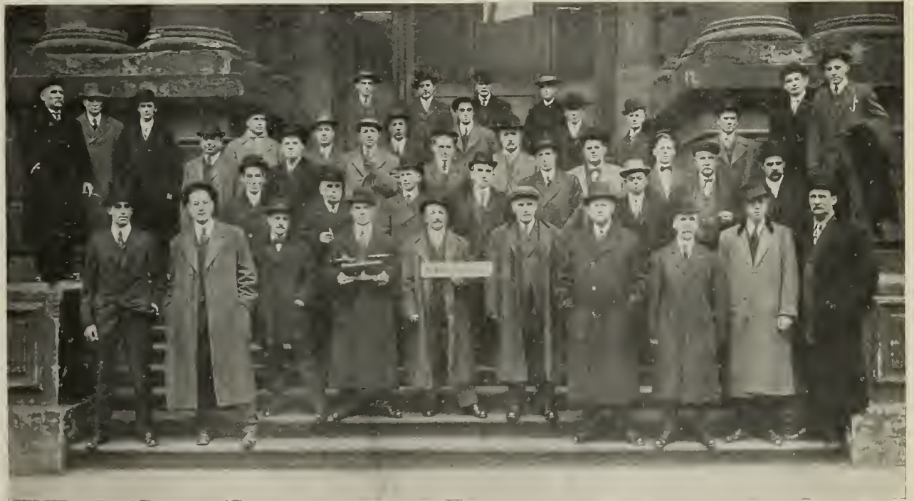
MEMBERS OF THE WEIGHING DEPARTMENT, MERCHANTS' EXCHANGE, ST. LOUIS, MO.
